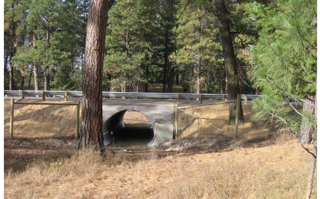
Figure 49. Wildlife Crossing Culvert Near Kalispell, Montana on Secondary Road 206. Photo Courtesy of Pat Basting.
